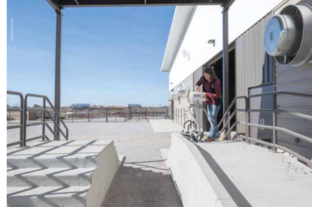
Hannah Bilovesky, NMSU equine instructor and equestrian team coach, demonstrates the handicap lift on the new permanent, equine-assisted therapy ADA ramp at the facility.
